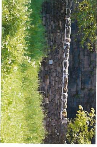
↓ (3) REGUILT A SECTION OF BOUNDARY WALL - FROM FIELD & FROM BARNSELEY ROAD (AFTER!)
