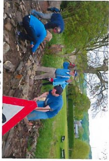
↓ (3) WALLING COURSE & SECTION OF WALL REPAIRED BY VOLUNTEERS
